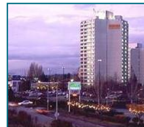
VANCOUVER AIRPORT CONFERENCE RESORT (RAMADA & PARK PLAZA TOWERS) $24 Million
